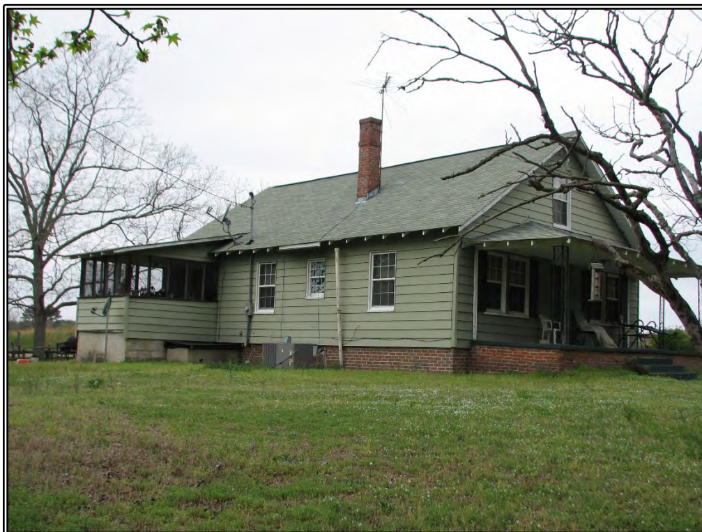
Figure 6. Photograph of Resource WA8360.1, southeast oblique.
